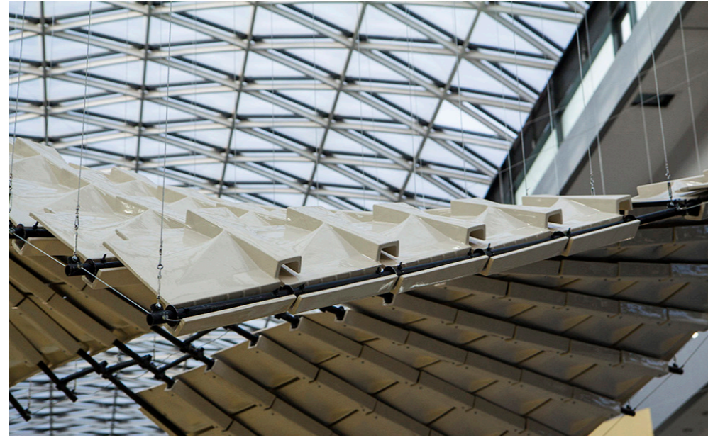
Digitally designed - traditional slip-cast production. Ceramic Shell , ceramic installation at the 2014 Cevissama, Spain. Material Processes and Systems Group at Harvard GSD. 1 Photo: Felix Raspall, 2014.
