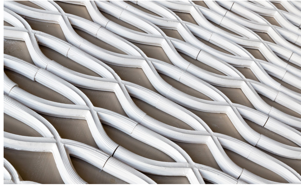
Digitally designed with deliberate tooling strategies - traditional slip-cast production. Chromosomes , screen wall exploiting tooling strategies for surface articulation of columnar tile structures. Material Practice as Research, Harvard GSD Fall 2014 course. 2 Photo: Harvard Graduate School of Design - Maggie Janik, 2014.
